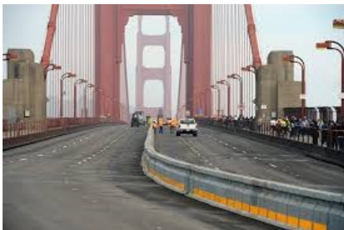
The new “zipper” MEDIAN on the Golden Gate Bridge
